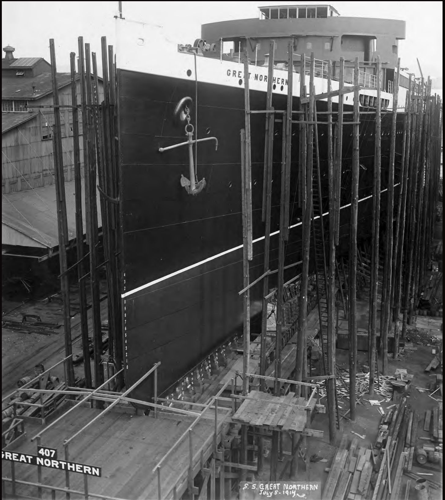
The bow of the Great Northern two days before her launch in Philadelphia. Shipbuilder Cramp & Sons numbered each of its ship hulls in succession. The Great Northern was No. 407 and the Northern Pacific was No. 408. Designed much like a yacht, the vessel's hull lines were so fine that they were described as "like a carving knife on edge." CRMM 411-9432
