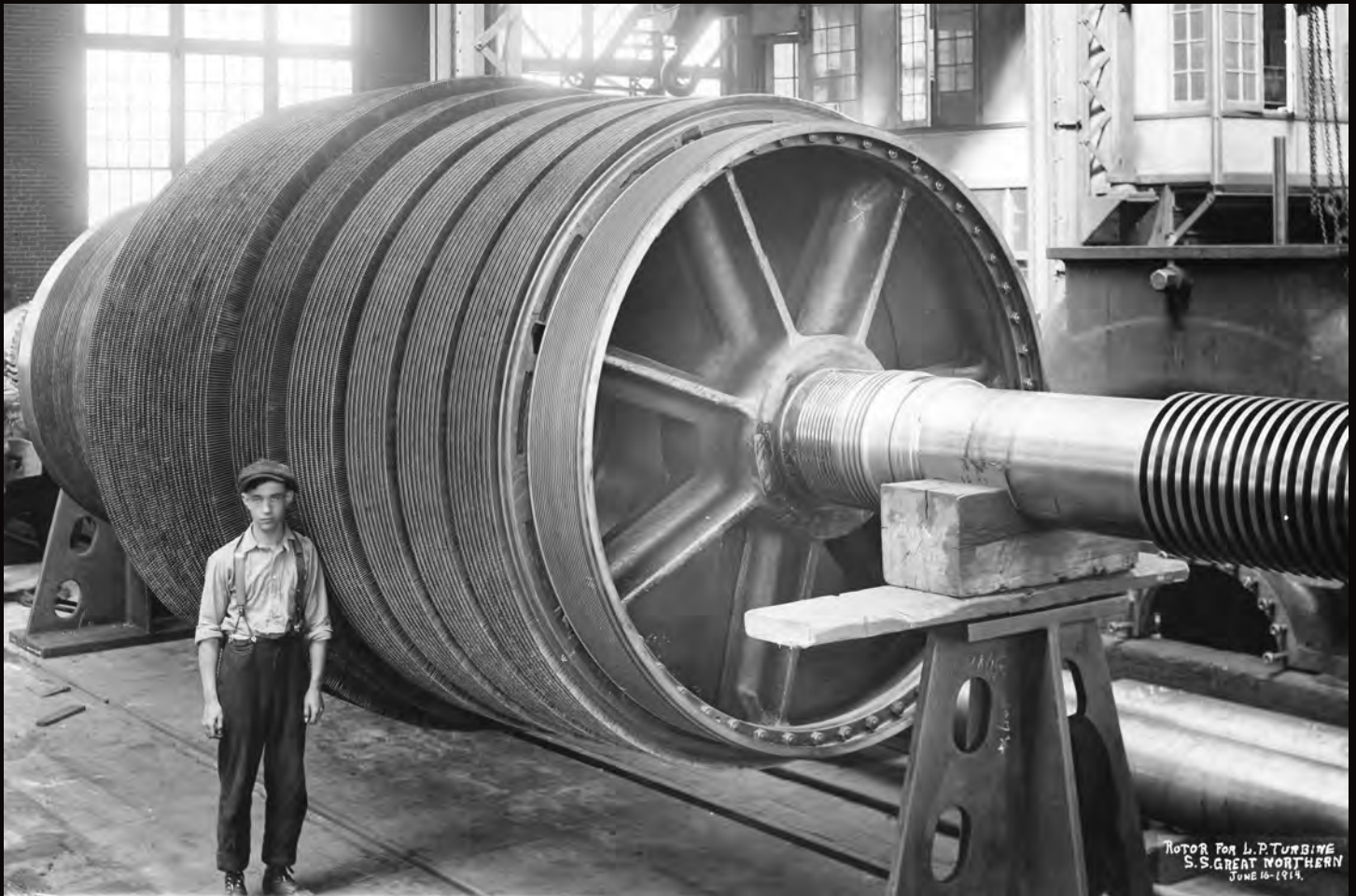
The huge size of the rotor for each Parsons turbine engine installed aboard the S.S. Great Northern is shown above with a shipyard worker in the foreground. This photograph was taken just three weeks before the vessel's launch on July 7, 1914. CRMM 411-9400
